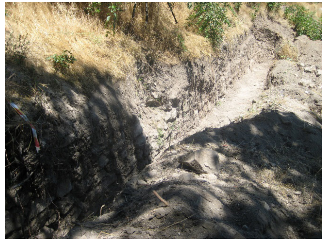
Fig. 28. Ottoman retaining wall.
