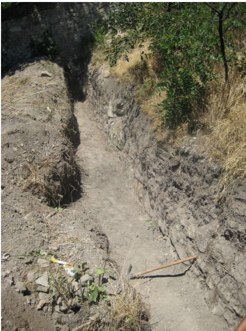
Fig. 29. Ottoman retaining wall.
