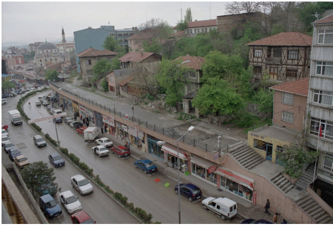
Fig. 5. Akpınar Neighborhood and municipality shops.
