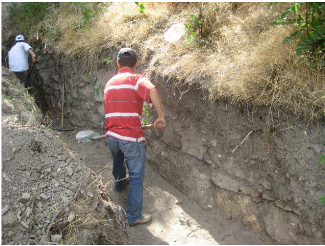
Fig. 27. Ottoman retaining wall works.
