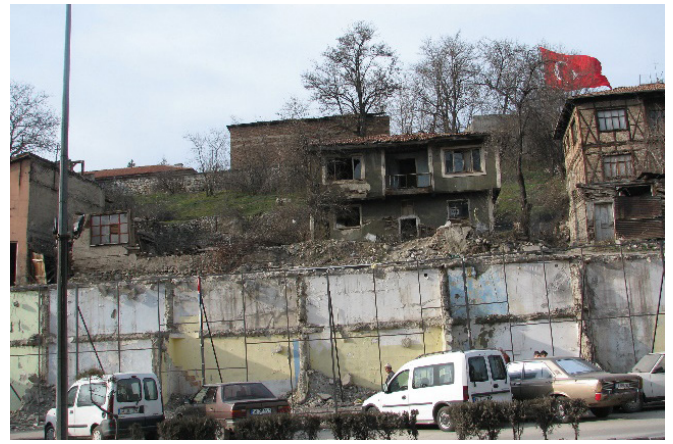
Fig. 6. Demolition of houses and shops.
