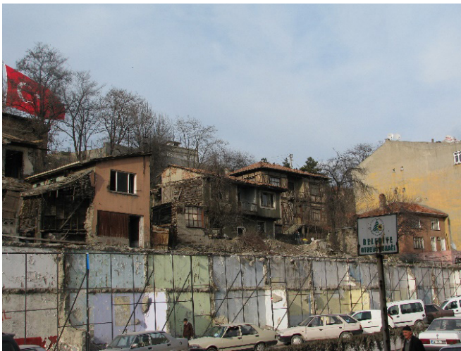
Fig. 7. Demolition of houses and shops.
