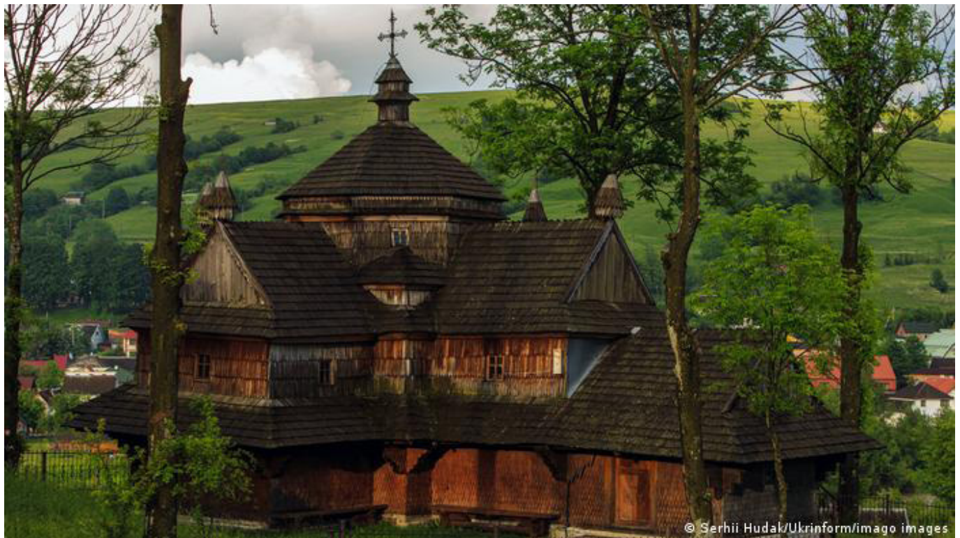
Fig. 5. Zakarpattia Oblast: Wooden tserkvas of the Carpathian Region. This UNESCO World Heritage Site is actually a series of 16 “tserkvas,” or churches, that are spread out over Poland and Ukraine in the mountainous Carpathian region. The wooden log structures were built between the 16th and 19th centuries by both Orthodox and Greek Catholic communities. They exemplify the timber-building tradition of Slavic countries, and their interiors are also quite renowned. https://www.dw.com/en/ukraine-rushes-to-save-cultural-heritage-from-destruction/a-61158291
